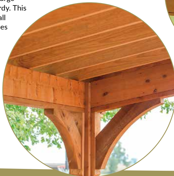
CEDAR SANTA FE Braces & Underside of Roof
